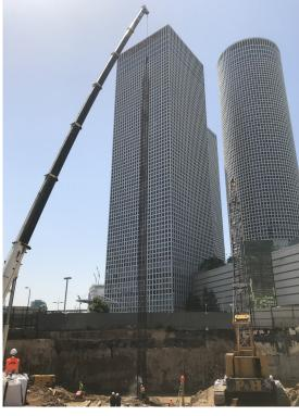
Pile reinforcement installation with O-cell assembly.
