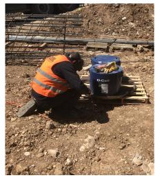
Assembly of the O-cell assembly
